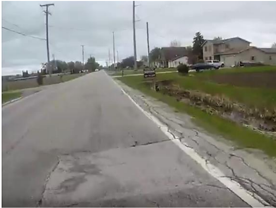
Figure 1: Before Construction (at Schwab Road Looking South)
